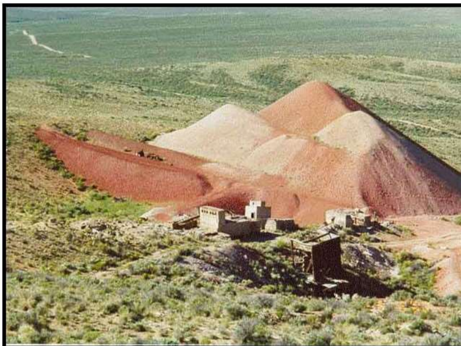
Figure 31. View of the Opalite mine processing plant and burnt ore pile (after Anderson 2003).
