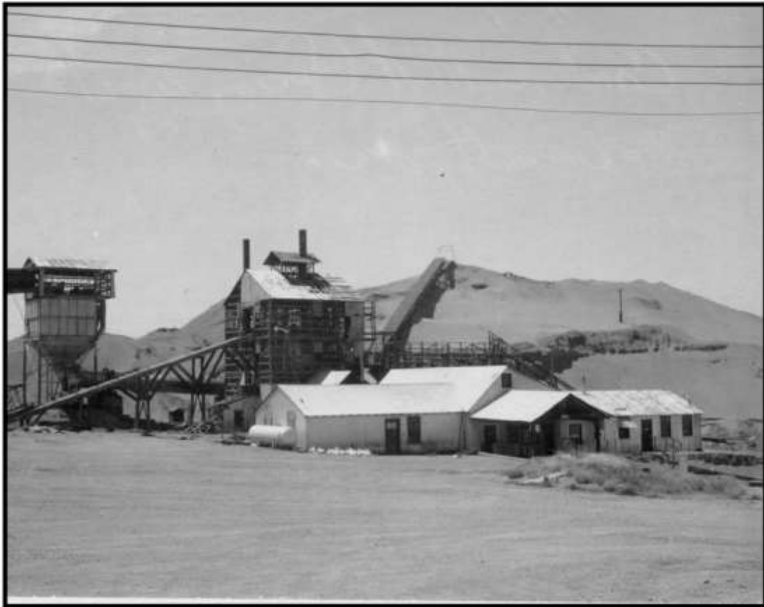
Figure 21. Abandoned Cordero mine processing facility in about 1980 (Placer Amex Staff circa 1980). The tall structure at center housed a Herschhoff multiple-hearth furnace. In 2011, following a site closure and cleanup project, all that remained on site was the calcines pile and the cylindrical body of the multiple-hearth furnace.
