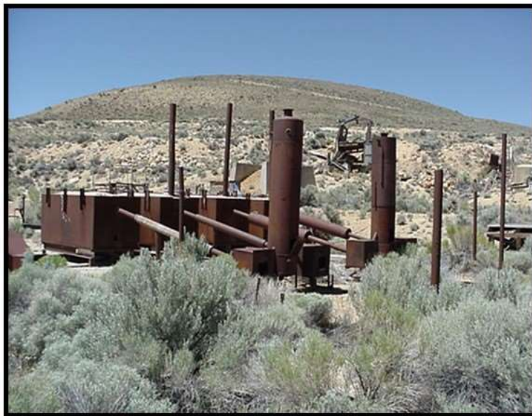
Figure 29. View of the Bretz mine retort configuration (after Anderson 2003).
