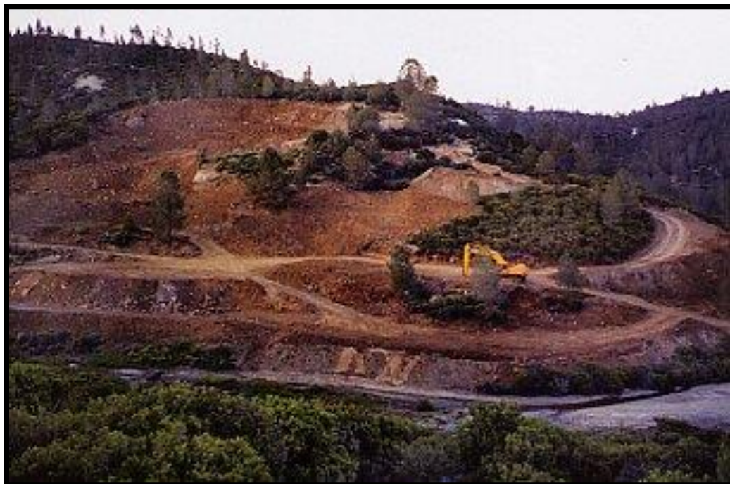
Figure 25. The Dallas Gem mine during 2006 near the end of excavation and gem stone recovery (after Wilson, 2008).
